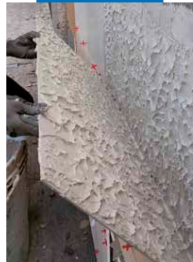
Checking the back face of the tile if it is completely buttered when laying on an external façade
