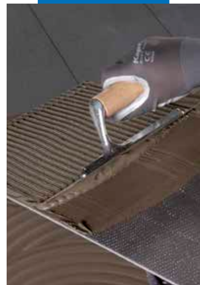
Spreading the adhesive on the back of the tile
