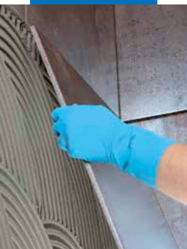
Laying large-sized tiles on walls
