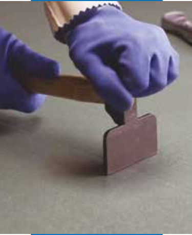
Pressing down the junction between sheets
