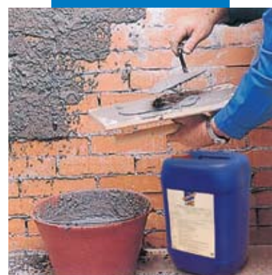
Spatter - dash coat modified with Planicrete SP
