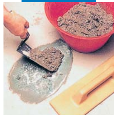
Floor patching: application of mortar
