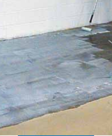
Application of Mapeprim SP
