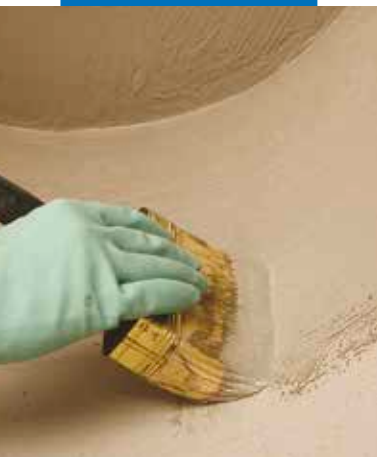
Waterproofing of details by brush
