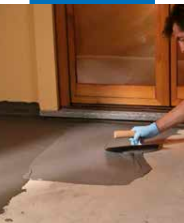
Waterproofing of terraces by trowel
