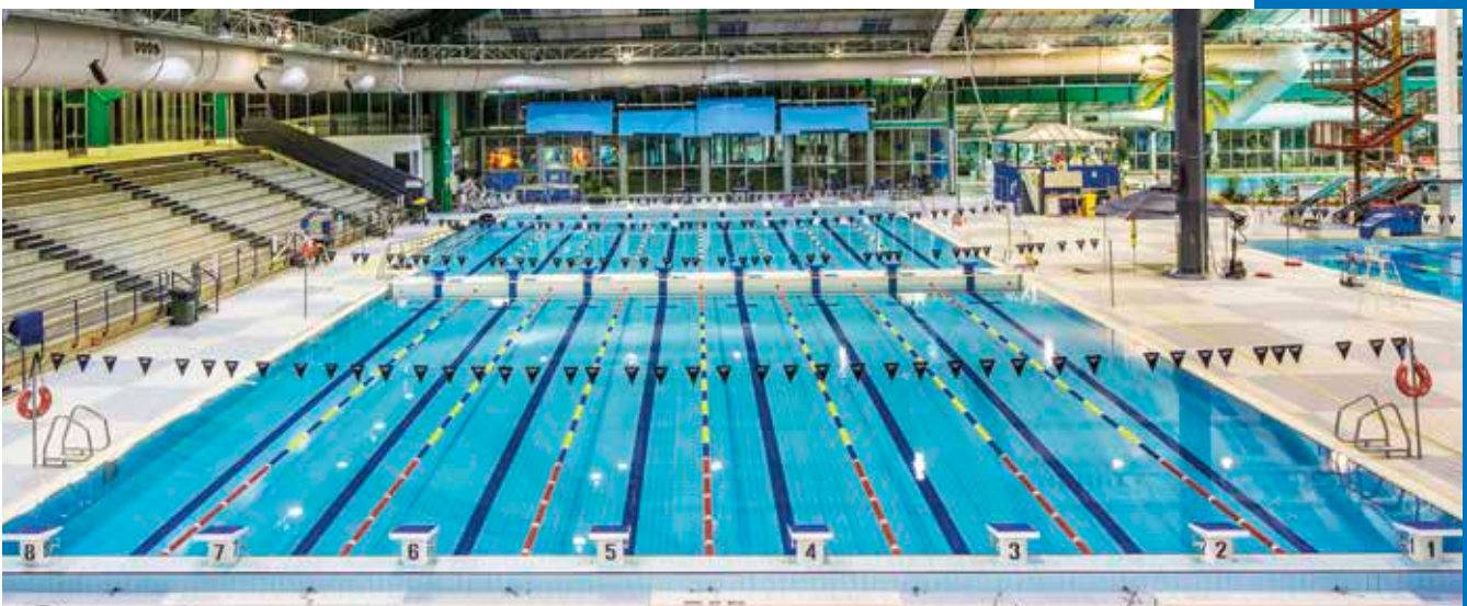
Completed 50m pool at the Adelaide Aquatic Centre
