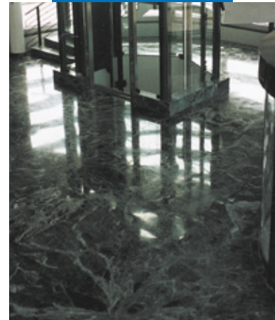
Verde Alpi green marble flooring in the Rolex building hall (Bienne - Switzerland)
