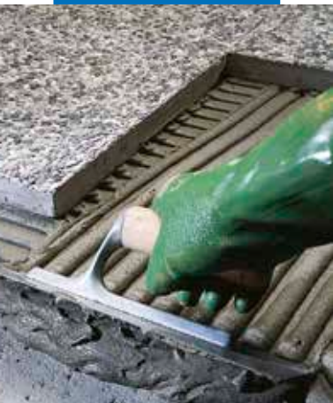
External installation of relief terrazzo "graniglie" tiles
