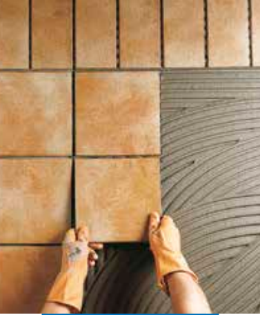
External installation of klinker tiles
